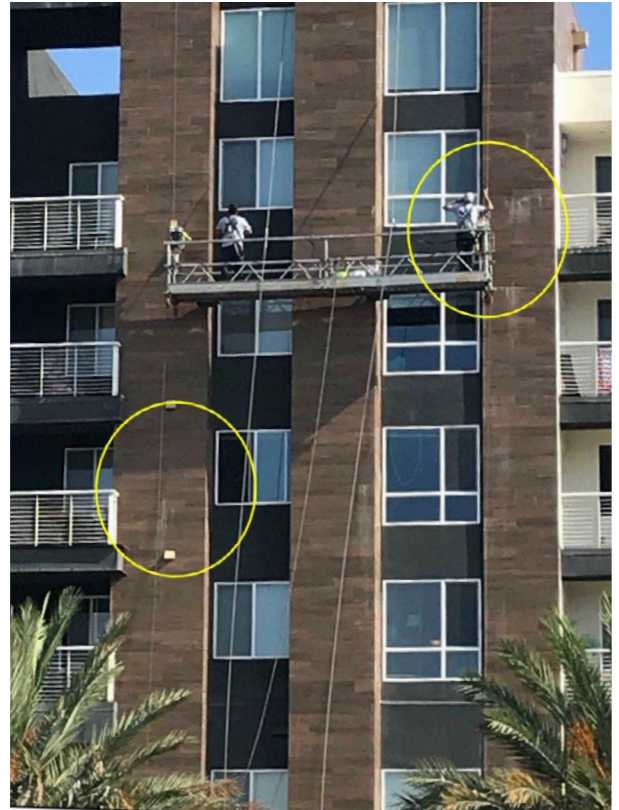
Removing Efflorescence
