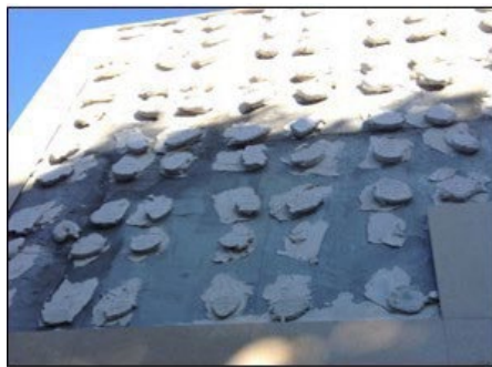
Spot-Bonding — Not an acceptable practice for ceramic, thin brick or dimension stone tile using ANSI A108 methods.
